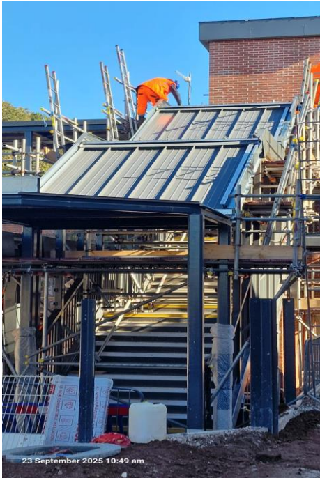
STAIRWAY ROOF CLADDING
