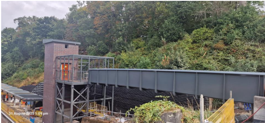
P2 LINK BRIDGE INSTALLED
