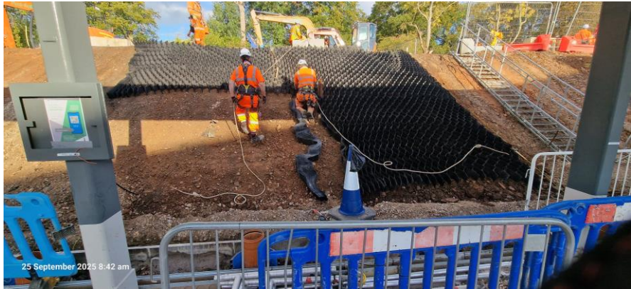
EMBANKMENT GEO-CELL
