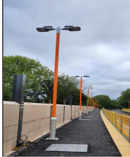
LC LAMP HEADS INSTALLED
