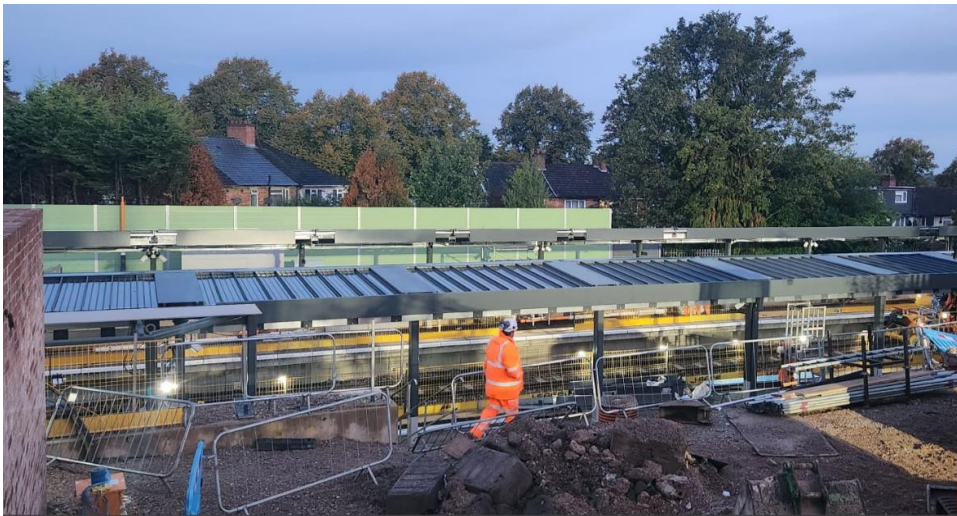
P1 CANOPY CLADDING COMPLETE
